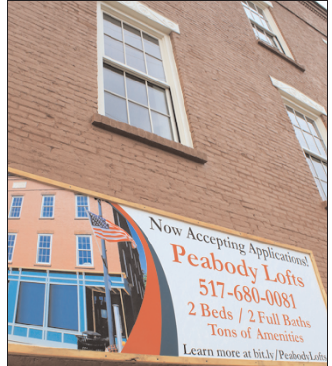
Bill Dobbins, president and CEO of Caster Concepts, has been striving to rebuild the Albion community. One way Dobbins has managed to do this is by purchasing and restoring the Peabody Building, which is located at 400 S. Superior St. in Albion, and creating several new businesses that are or will be located inside, including the Peabody Lofts. (Photo by John Hendler)
