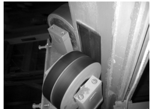
Floor-to-floor elevator guide wheel of NYTEC-HS
